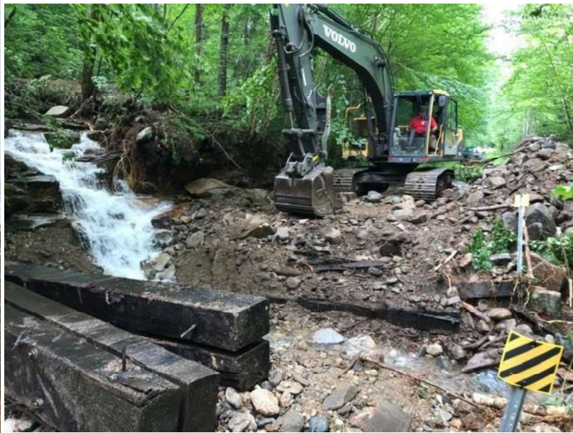
Repair and construction on Presidential Rail Trail
